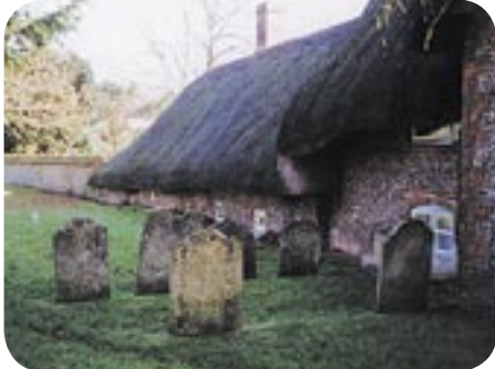
Vernacular building materials including long straw thatch at Gable Cottage
