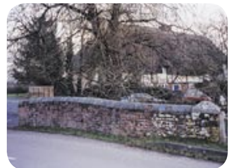
Brick abutments over the river crossing at Stoke
