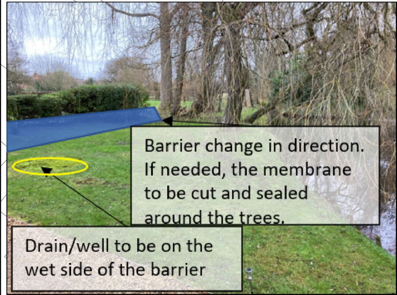
PHOTO B: BARRIER CHANGE IN DIRECTION AT NORTH CORNER OF THE LODGE. THE PHOTO SHOWS THE DRAIN / WELL LOCATION
